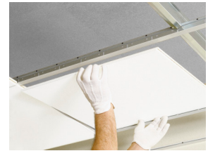
The individual tiles are easily demountable
