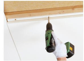
Master F is installed by screw fixing
