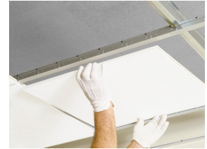
The individual tiles are easily demountable
