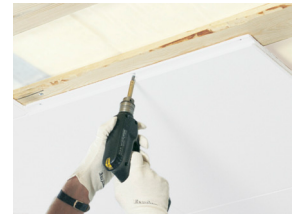
Focus F is installed by screw fixing
