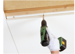
Master F is installed by screw fixing
