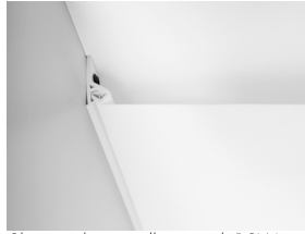
Clipso ceiling installation with PCW profile.
