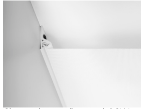
Clipso ceiling installation with PCW profile.
