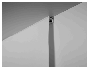
Clipso wall installation with PCC profile.
