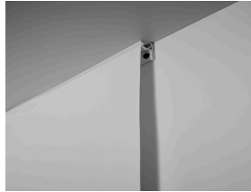
Clipso wall installation with PCC profile.
