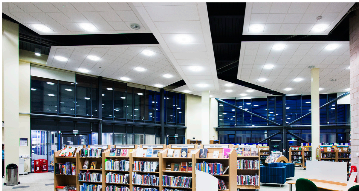
Seaham Contact Centre, Seaham, United Kingdom
