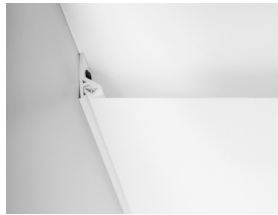
Clipso ceiling installation with PCW profile.
