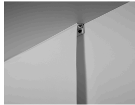
Clipso wall installation with PCC profile.
