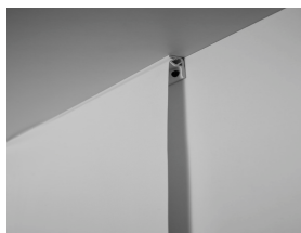
Clipso wall installation with PCC profile.
