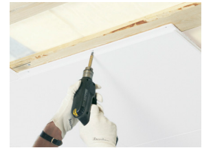
Focus F is installed by screw fixing
