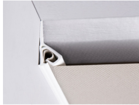
Clipso ceiling installation with PCW profile.
