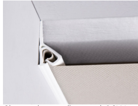
Clipso ceiling installation with PCW profile.
