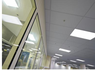
Macana Construction specialise in high care environments so therefore chose Ecophon Focus due to the excellent sound absorption and for applications where an attractive suspended ceiling is required where easy removal of individual tiles is essential. Ecophon Focus E has a recessed visible grid and a tegular edge design, creating a ceiling with a shadow effect that accentuates each tile and partially conceals the grid system.
