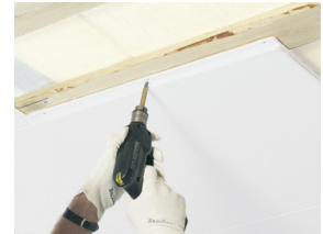
Focus F is installed by screw fixing
