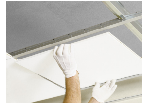
The individual tiles are easily demountable
